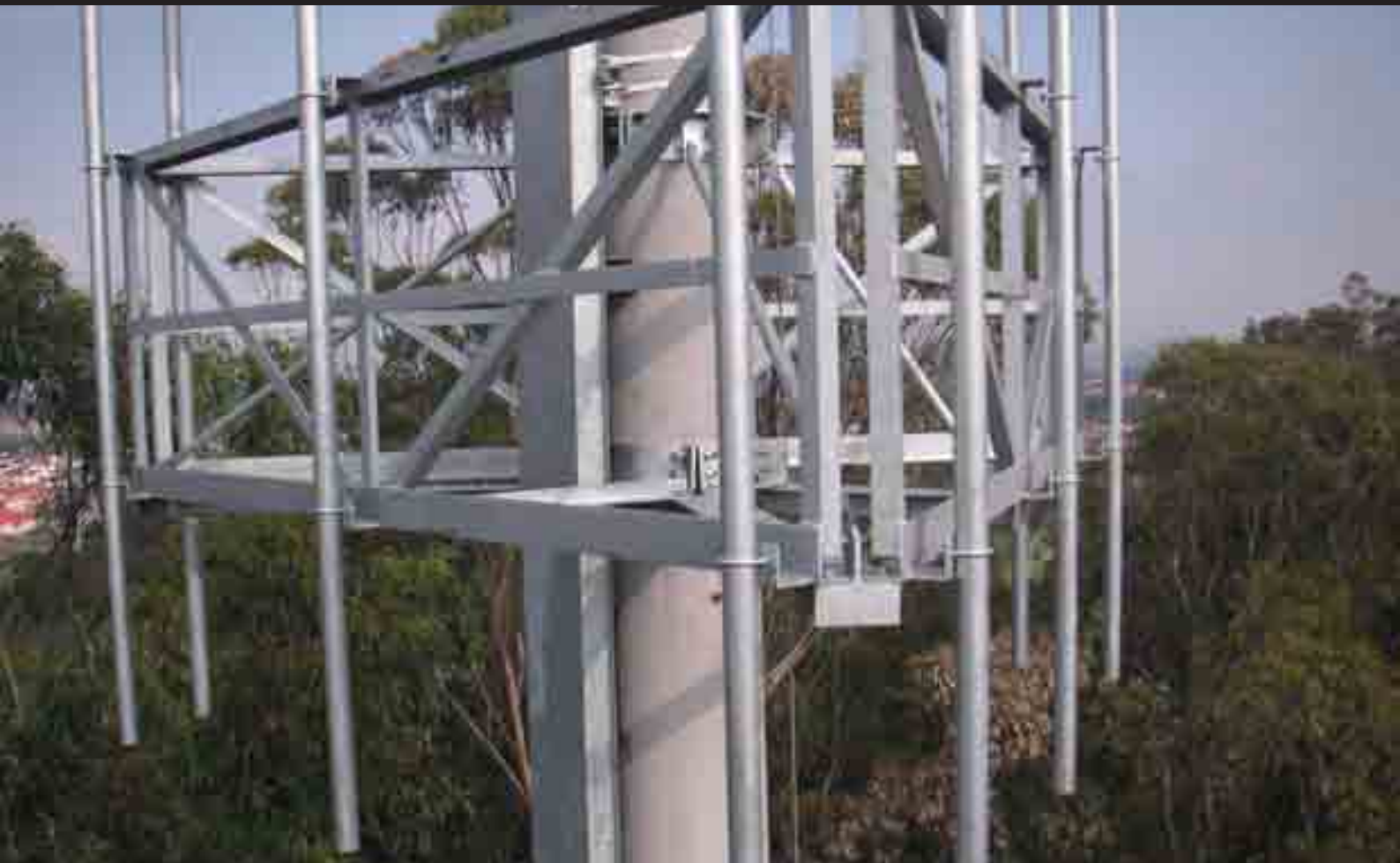
Head frame installation
