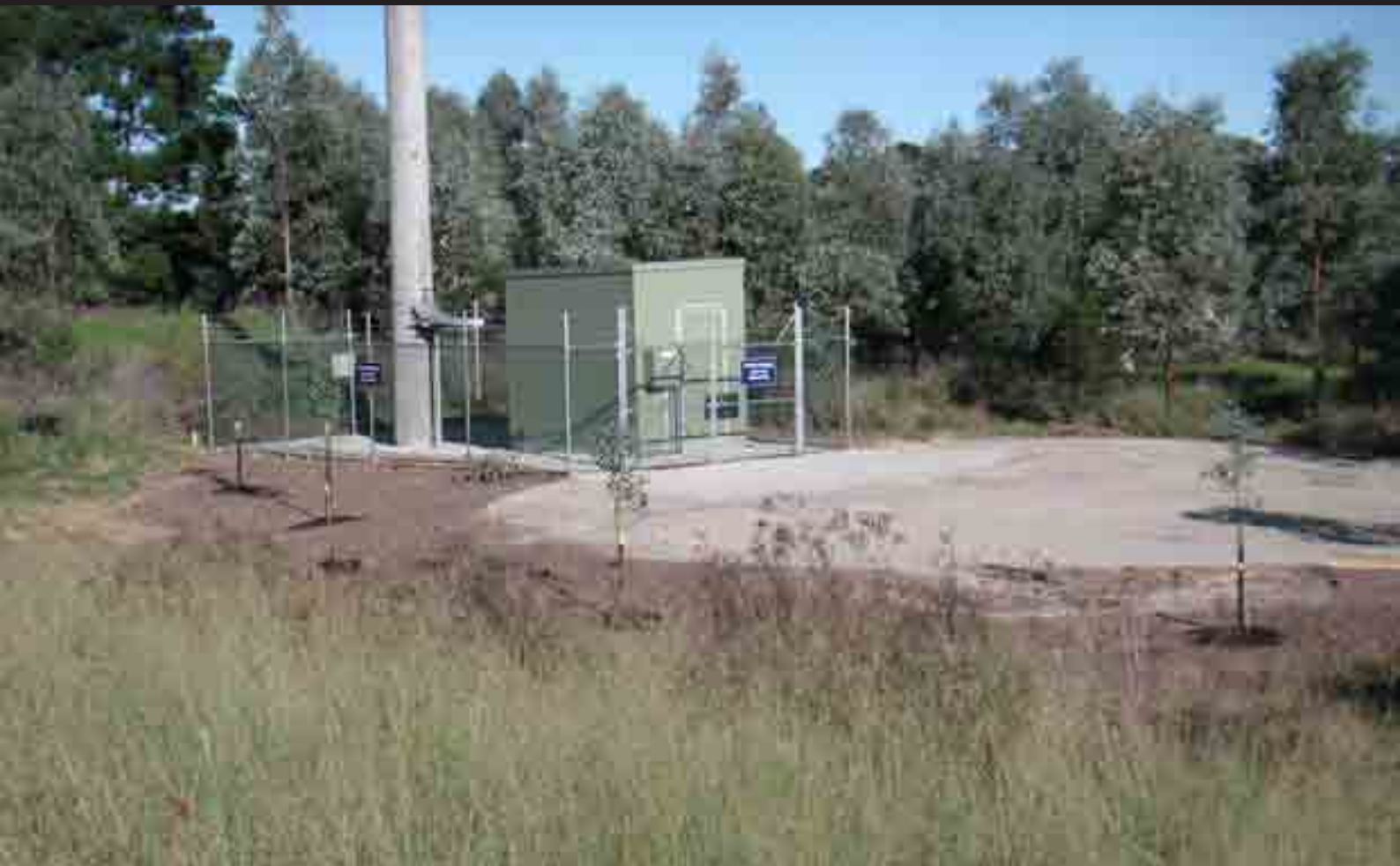
Telstra installation Roper Road
