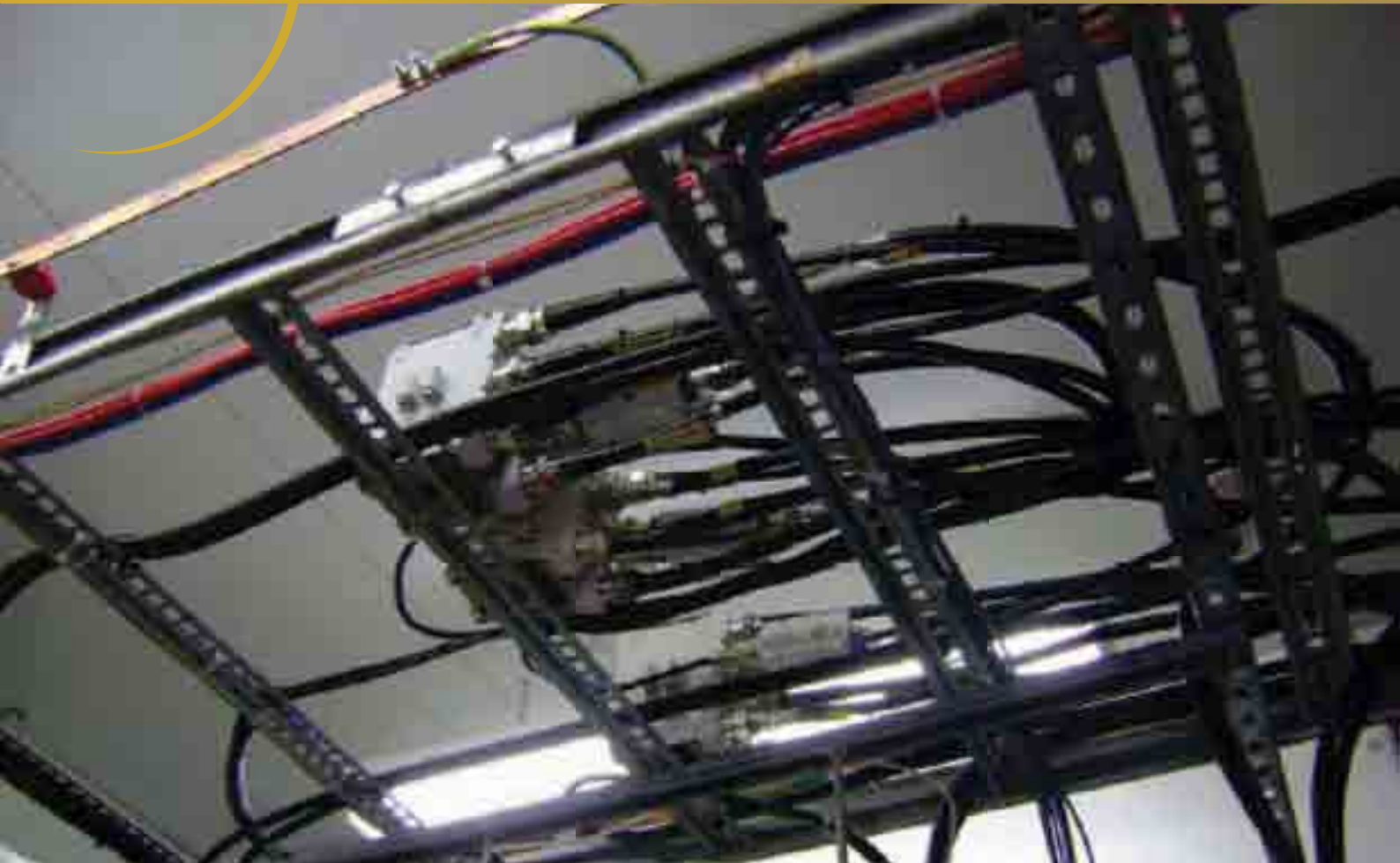
Diplexer and bias T install
