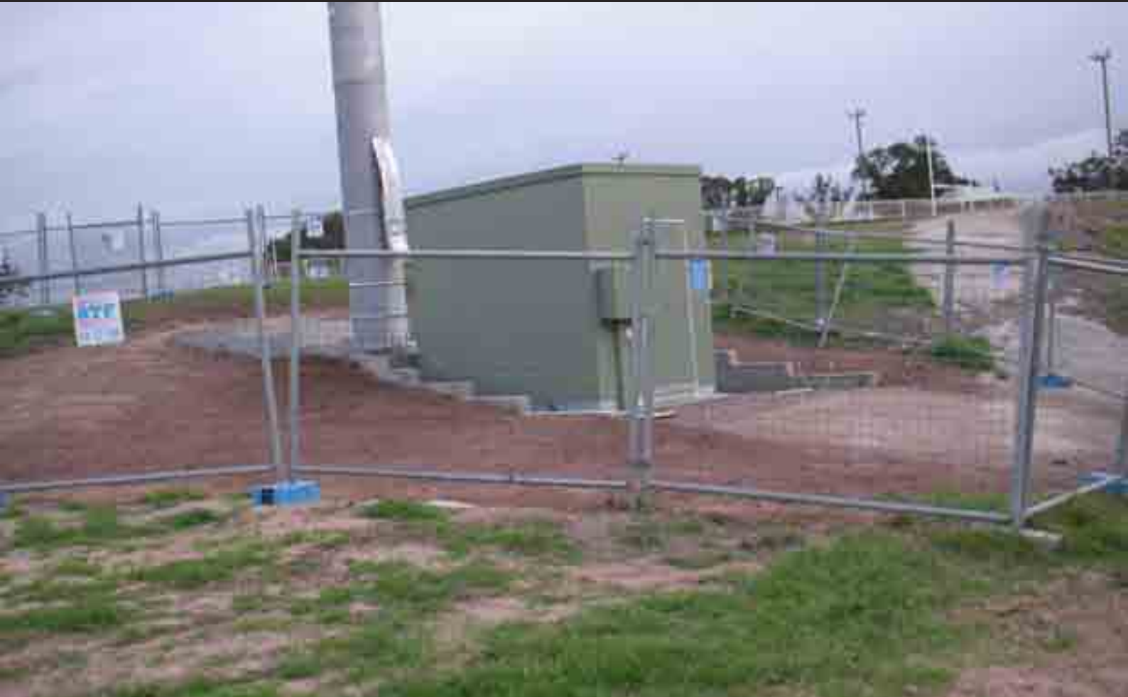
Full build for Telstra "Morpeth"
