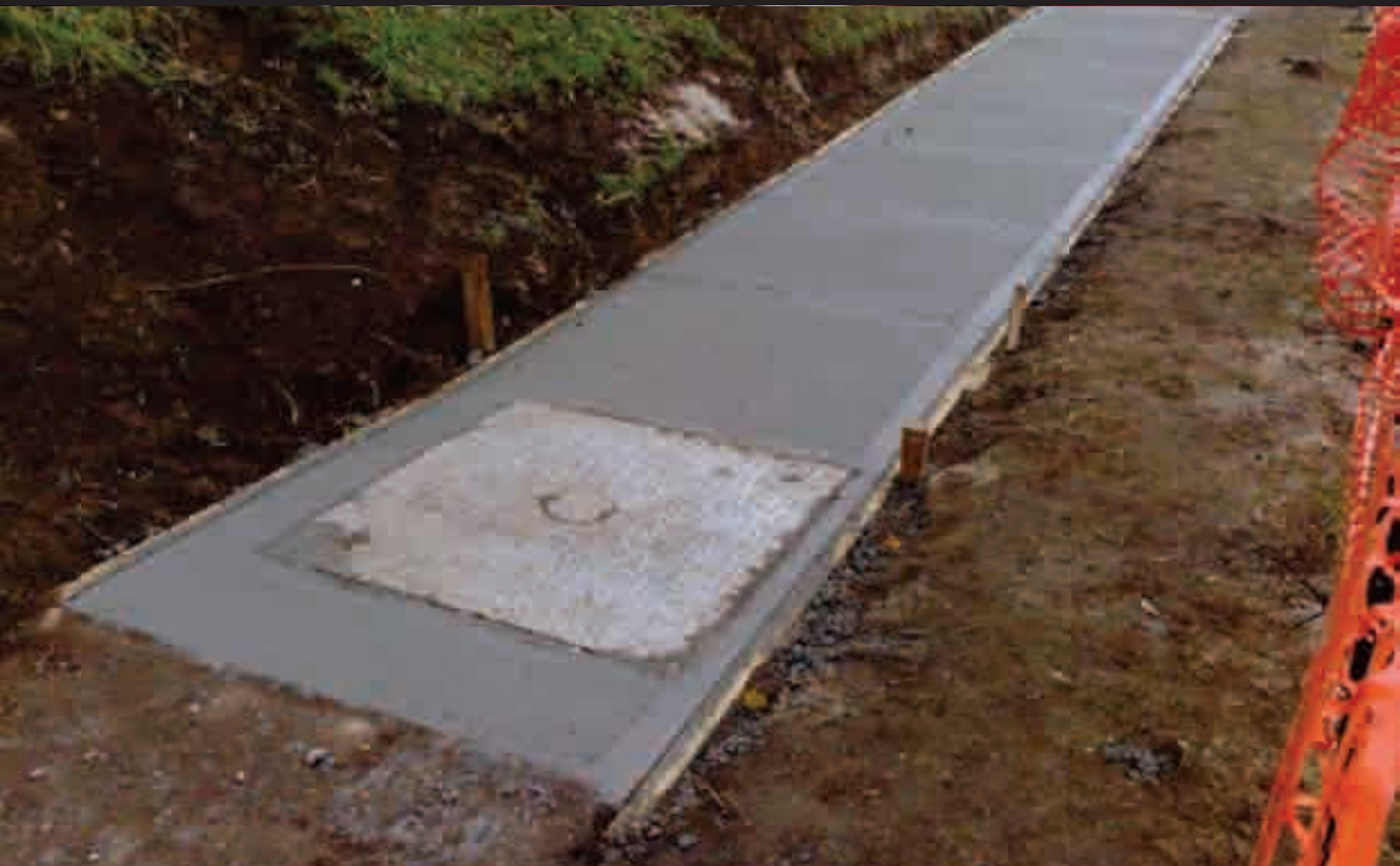
Underground cabling and concrete incasing
