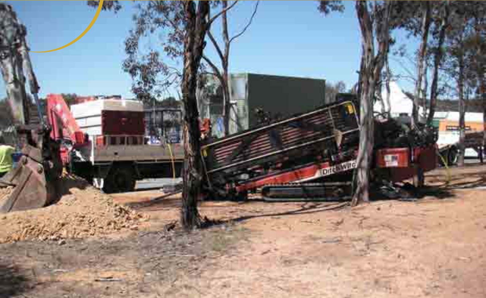
Under road boring
