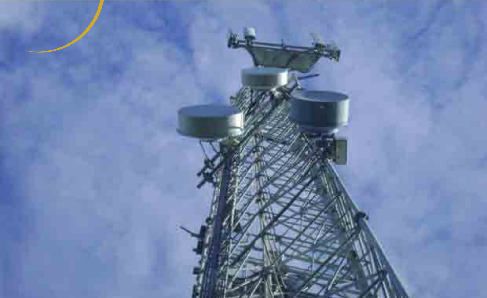
Face mount removal and upgrade
