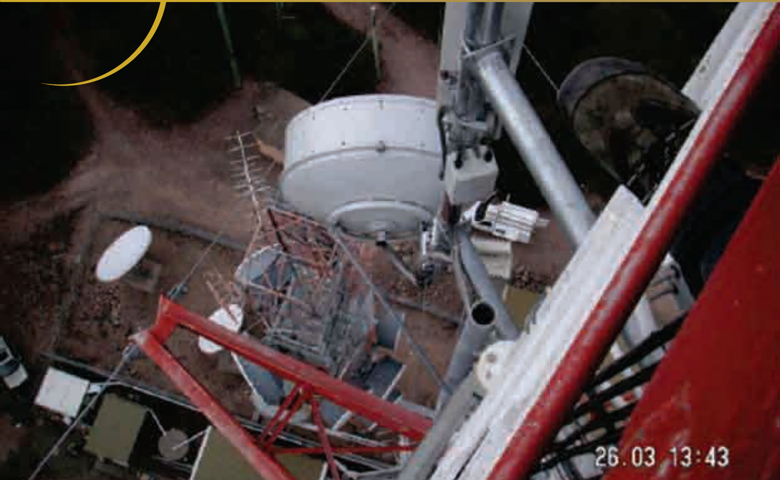
Radio and panel antenna install
