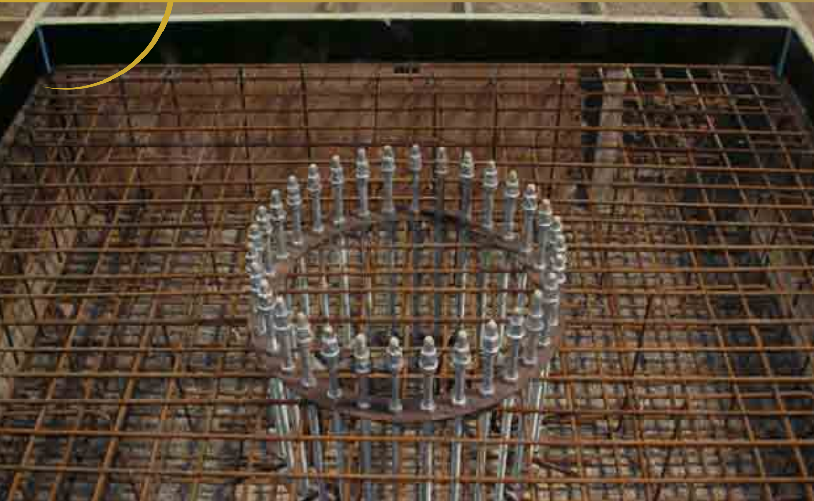
Pole footing M5
