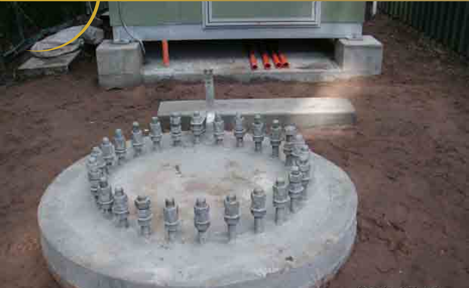
Shelter and pole foundation in water logged area
